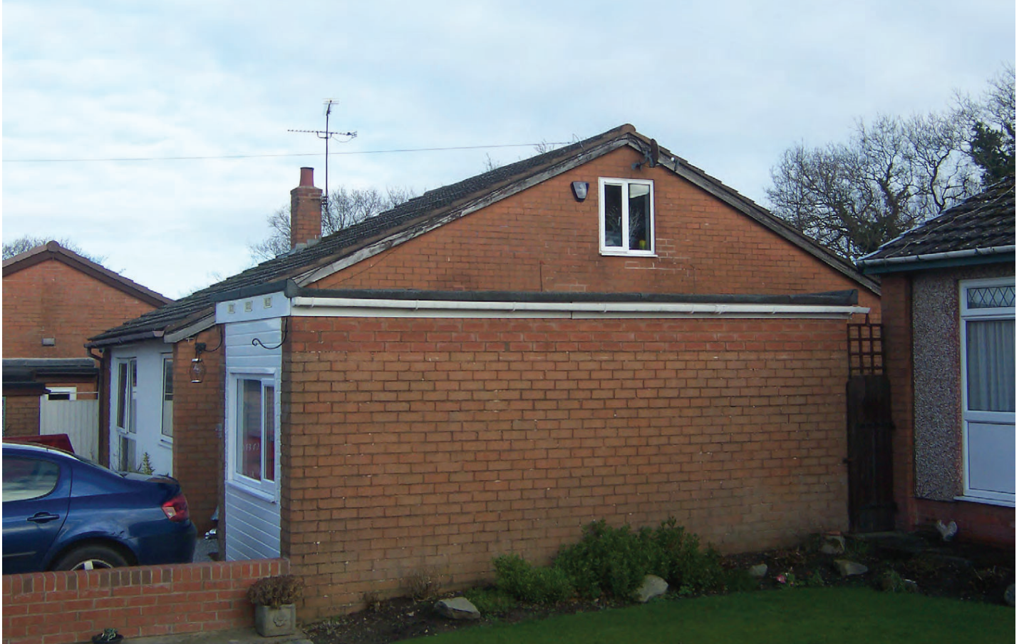
6.1 - 064256 Muirfield Road, Buckley
