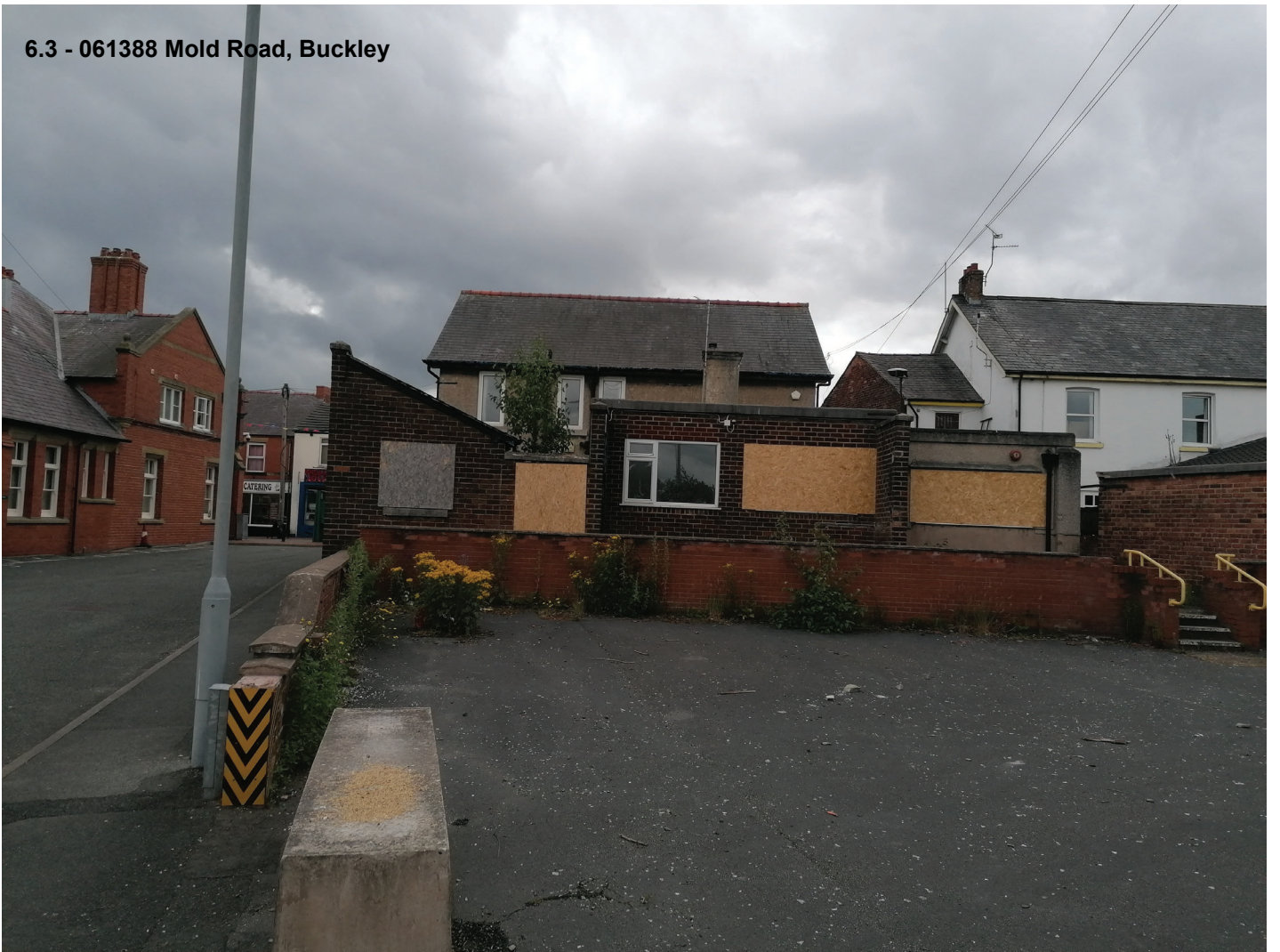
6.3 - 061388 Mold Road, Buckley
