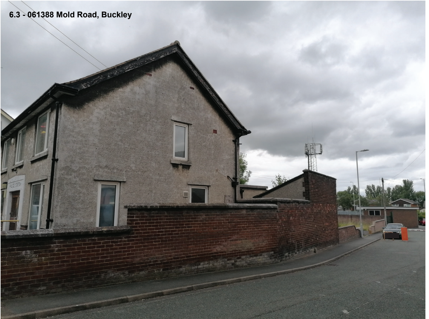
6.3 - 061388 Mold Road, Buckley
