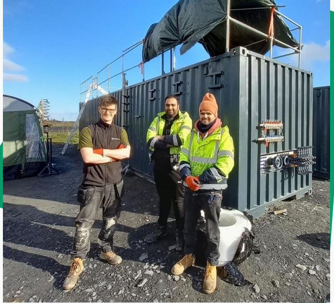
Three learners at Coleg Cambria, Llysfasi unveil the new Micro-Anaerobic Digestion (AD) system by Biofactory Energy
