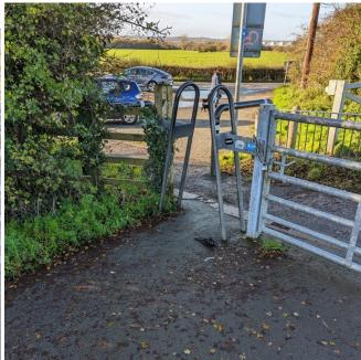
Barrier Type: Fixed A Frame Barrier adjacent to Gate
