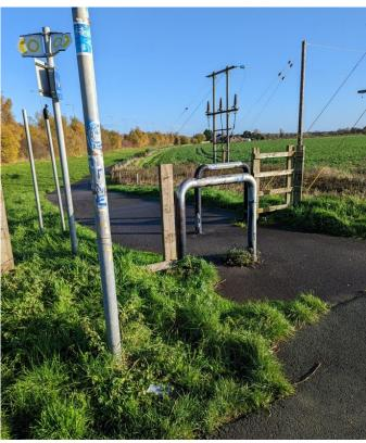
**Barrier Type: Chicane Barrier**
