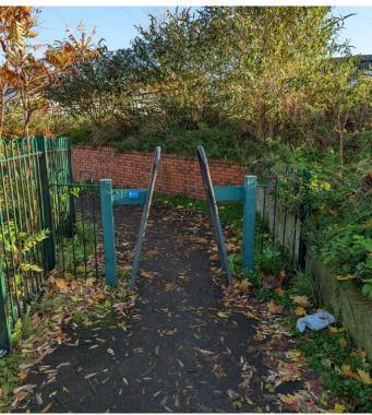
**Barrier Type: Fixed A Frame Barrier**
