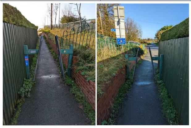
**Barrier Type: Fixed A Frame Barrier**
