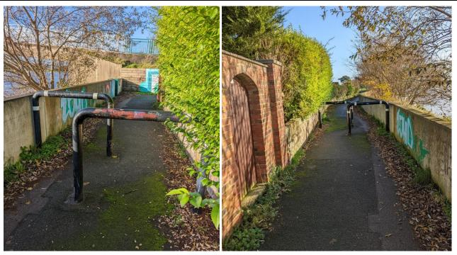
**Barrier Type: Chicane Barrier**
