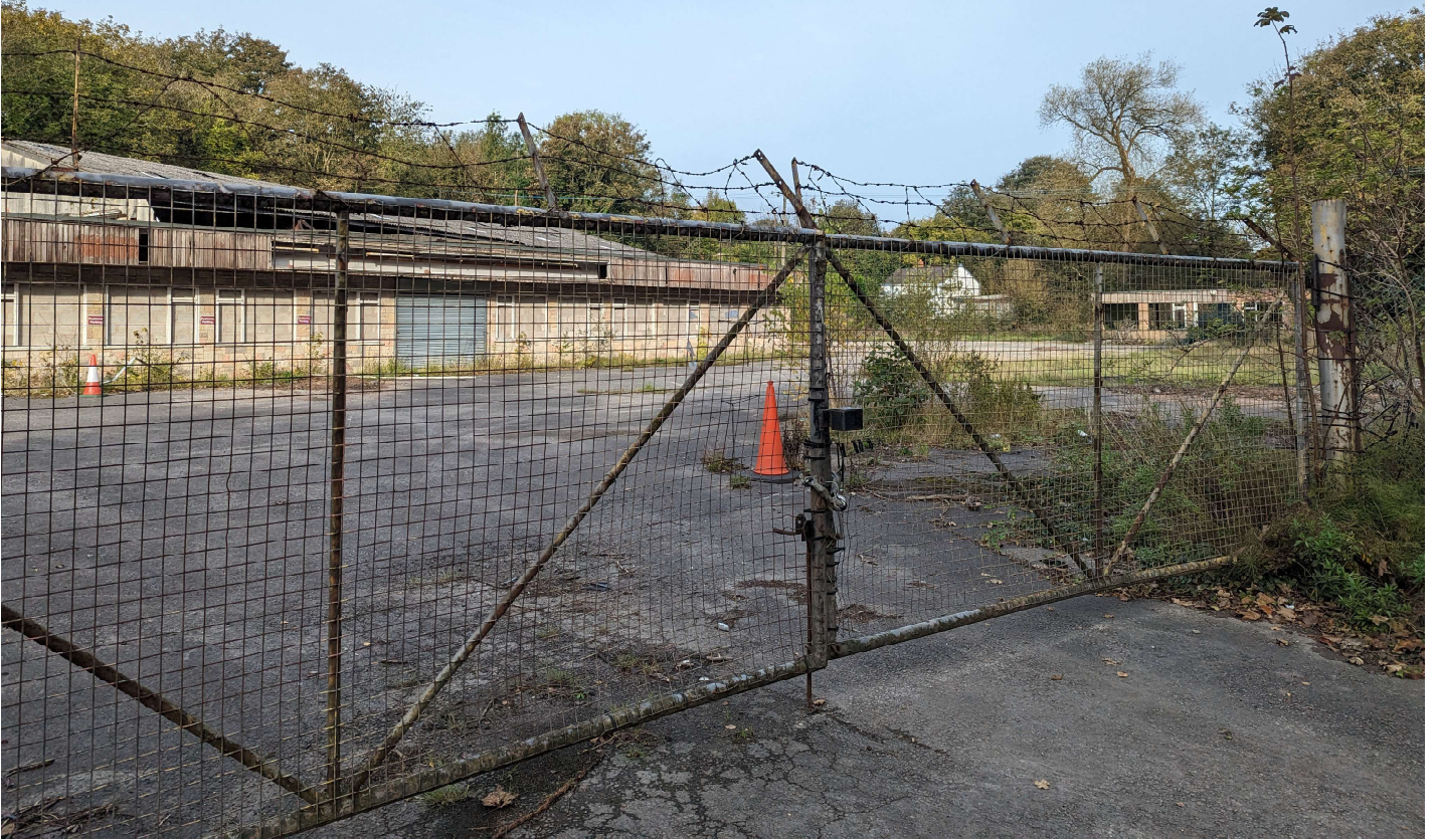
6.1 FUL/000001/23 - former Spectrum Garden Centre, Wrexham Road, Cefn-Y-Bedd
