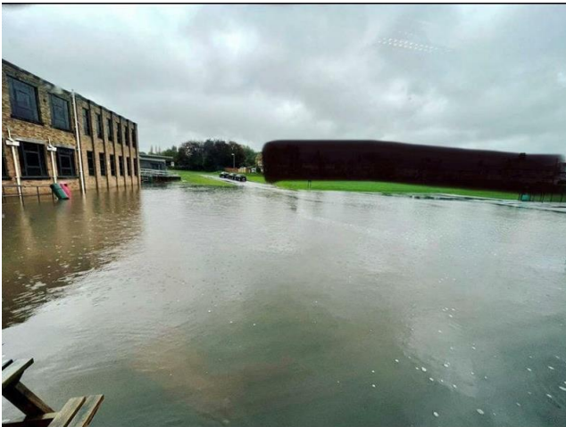
Figure 11: Flooding experienced in Flintshire School.
