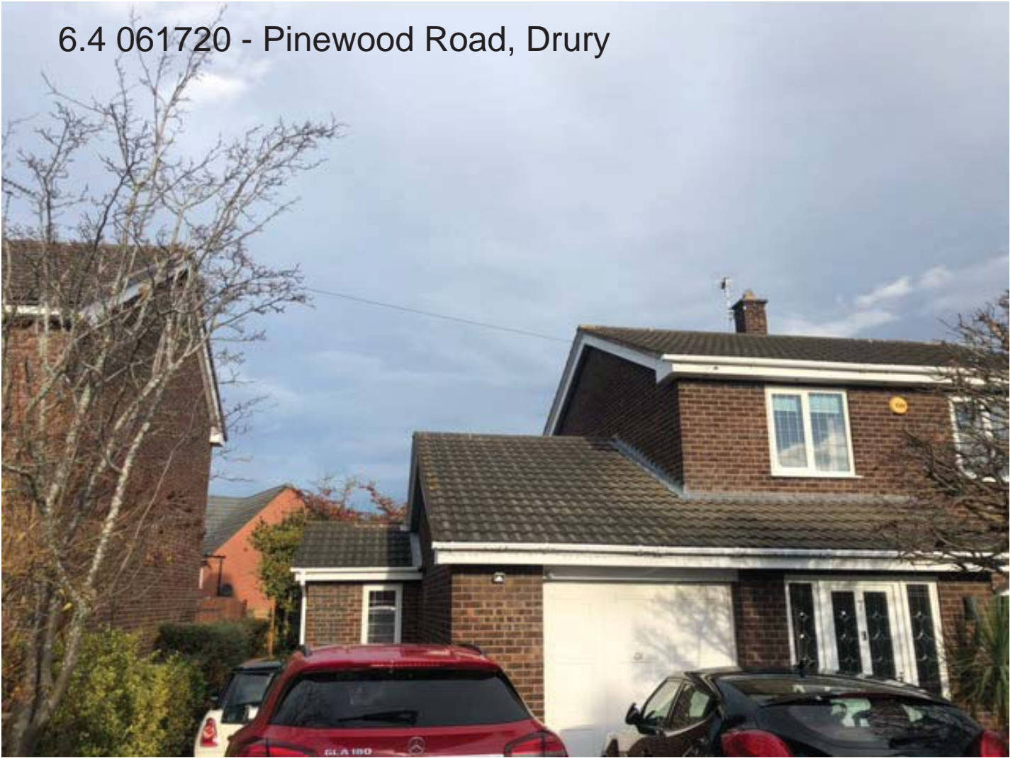
6.4 061720 - Pinewood Road, Drury
