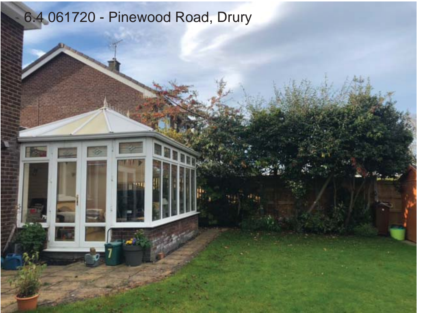
6.4 061720 - Pinewood Road, Drury
